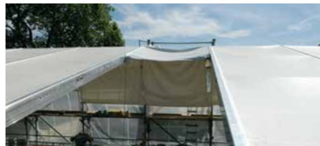
Temporarily open "empty bay" for servicing the site; the gaps between the frame sections are also very suitable for equalisation in a longitudinal direction
