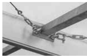
[02] Purlin + tensioning strap
